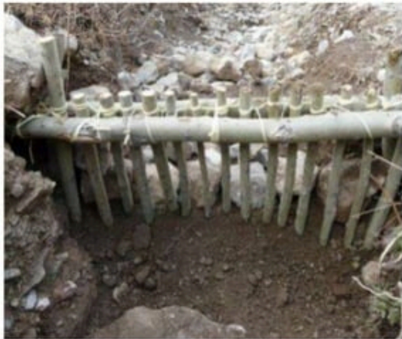
Palisades with double horizontal pole
