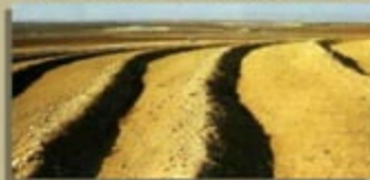
Construction of Contour Bunds
